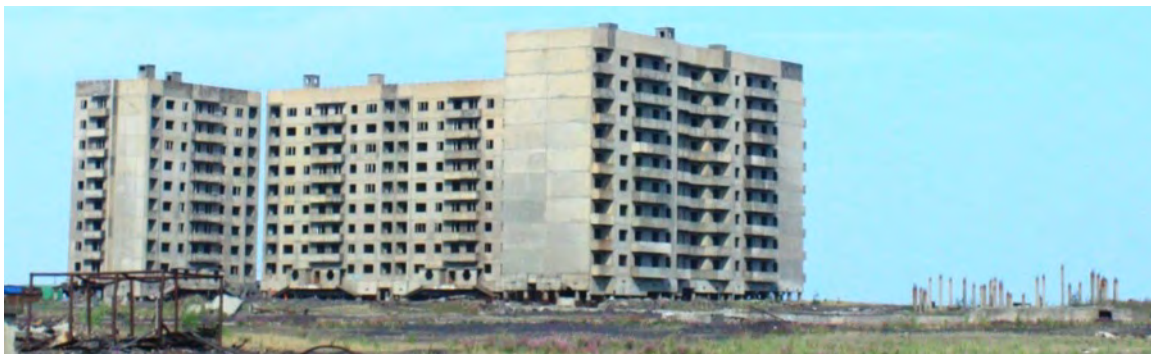
Figure 29. Building constructed using piling foundation on permafrost. The same type of piles can be seen on the right from the building. Various heights of the piles are the result of differential frost heave processes over the construction site. (Photo: D. Streletskiy, July 2013)
